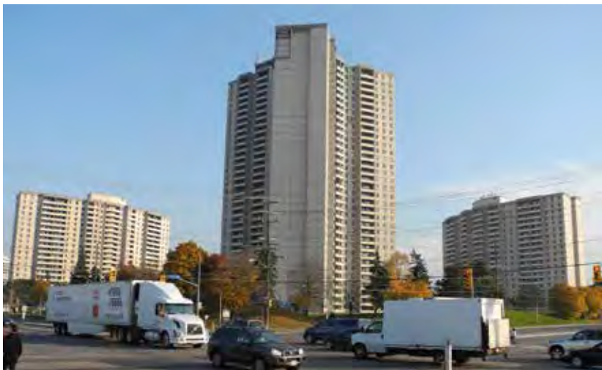
Figure 7 The Palisades building complex. “Somewhere to house them”. Is it a stockade that has shunted the marginalized into a suburban ghetto? Or is it a group of neighbourhoods with a strong sense of place and a commitment to community? Photograph courtesy of L. Anders Sandberg.
